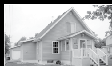
108 South Lincoln Street $85,000
